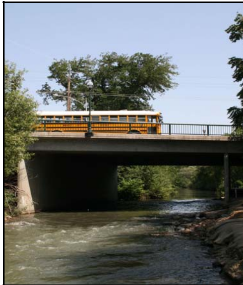
The G Street Bridge is one of the main arteries carrying north-south traffic.
