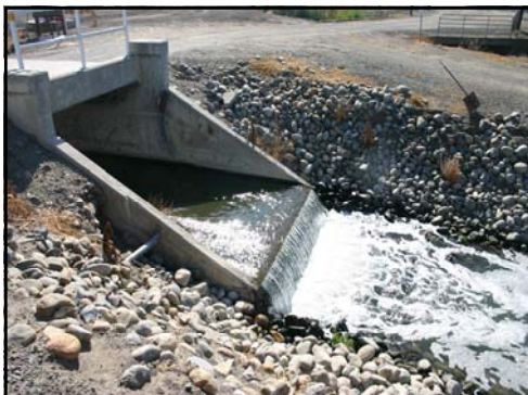
Upgrades to the City's wastewater treatment plant will improve the quality of water discharged back into the local environment.
