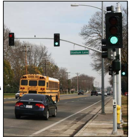
The new traffic signal at Yosemite Avenue and Stadium Lane.
