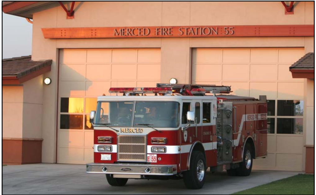
Fire Station 55 on Parsons Avenue was funded through City impact fees.
