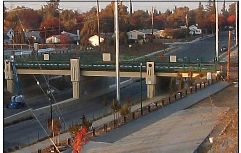
The G Street underpass before it was opened to the public.
