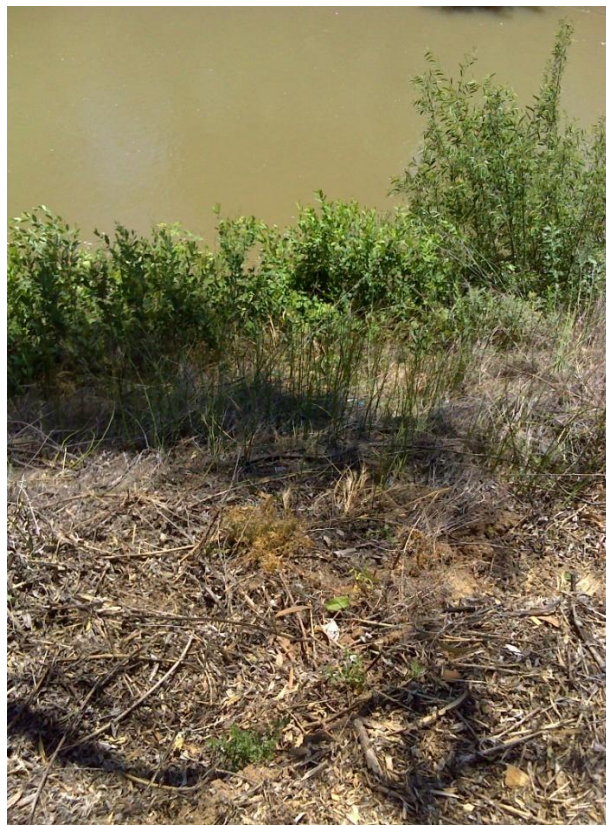
South view down the slope
