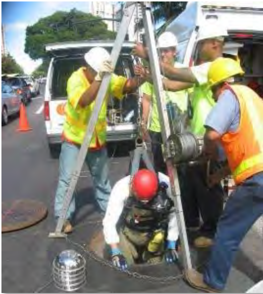
Photo 2-1. Confined Space Entry
