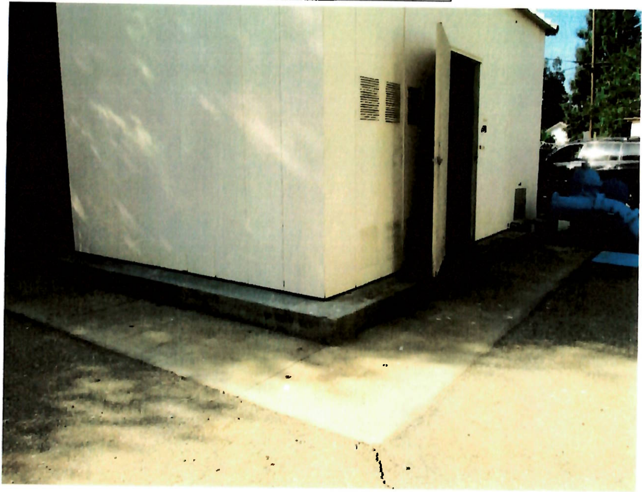
Well 7B Concrete Pad approximately 17' x 31'
